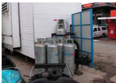
Secured to other cylinders
