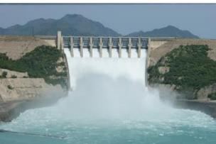
the sea level while it is 485 ft high from the riverbed. The resulting water reservoir lake has a total surface area of 250 square kilometers. Since its inception, it has played a vital role in irrigation, hydroelectric power generation as well as flood control for Pakistan.
